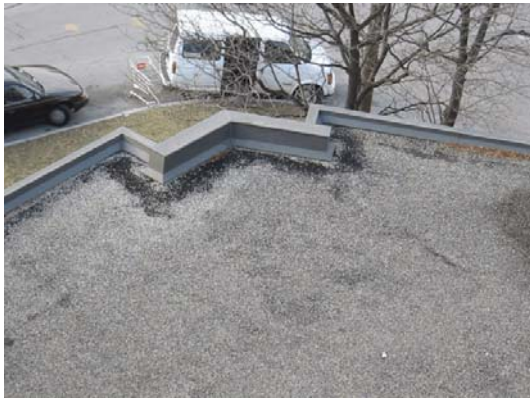
Figure 2: Convection heat loss from exterior wall/flat roof perimeter detail, due to lack of continuous wall/roof air barrier.
